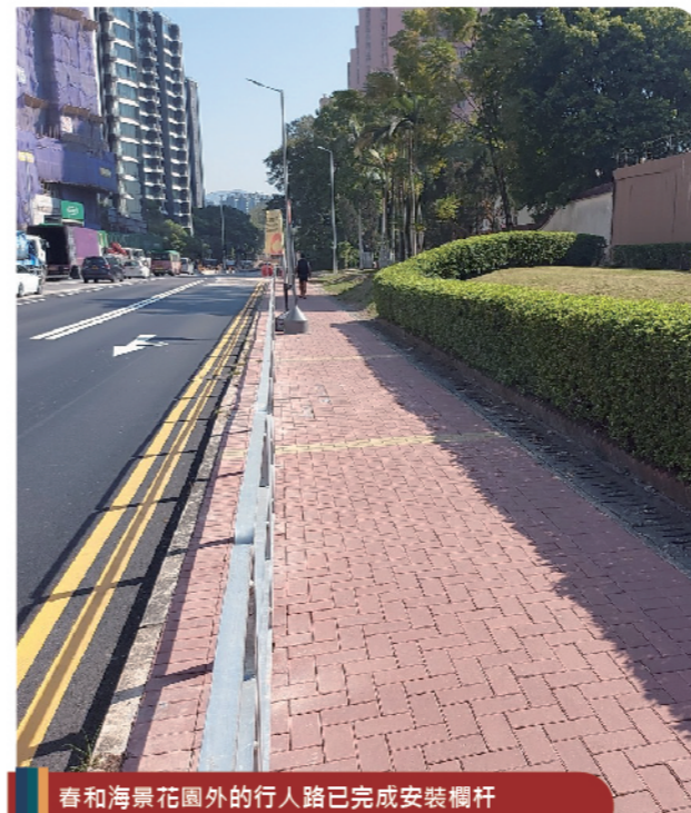
春和海景花園外的行人路已完成安裝欄杆 Completed installation of railing along footpath outside Spring Seaview Terrace
