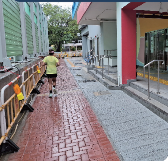
「齊+」@三聖過渡性房屋外鋪砌及修復行人路 Laying of paving blocks and reinstatement of footpath outside 'To + Gather' @ Sam Shing transitional housing
