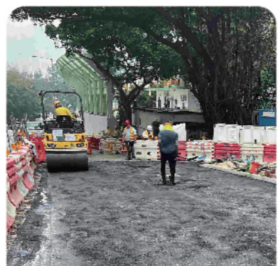
南岸附近鋪設瀝青 Laying bituminous material near South Crest
